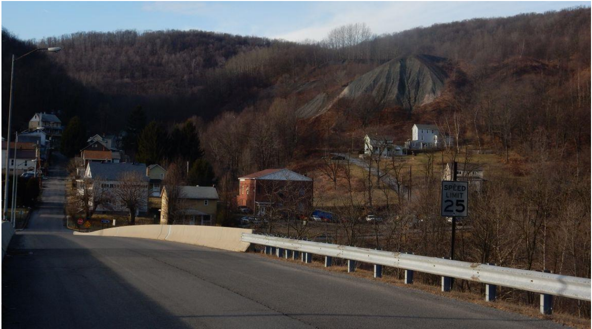
FIGURE 2.7 – COAL REFUSE PILE ABOVE EHRENFELD, PA
